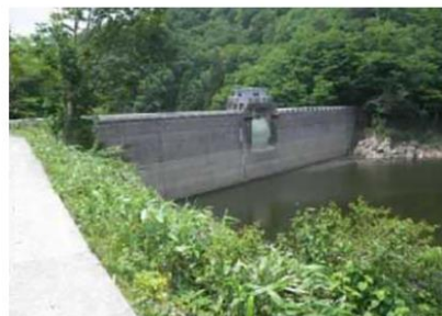
Nakatsu Dam (Photo taken from the official Tottori Prefecture web site)
