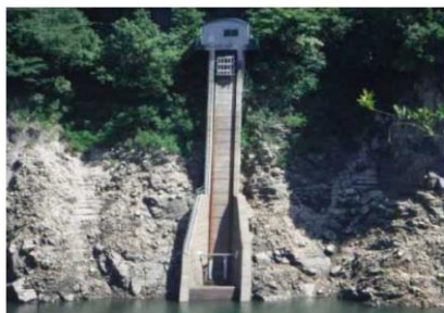
Hinogawa Daiichi Power Station (Photo taken from the official Tottori Prefecture web site)
