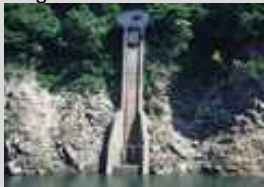
Hinogawa Daiichi Power Station
