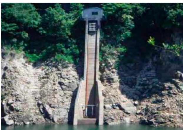
Hinogawa Daiichi Power Station (photo from the official website of Tottori Prefecture)
