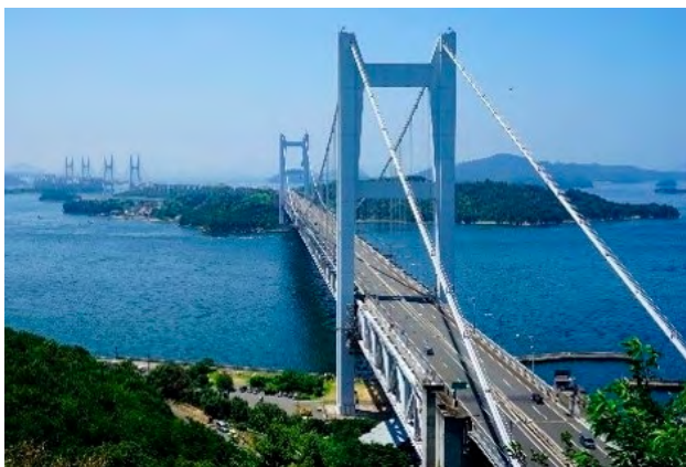
Seto Ohashi Bridge (Seto Chuo Expressway)
