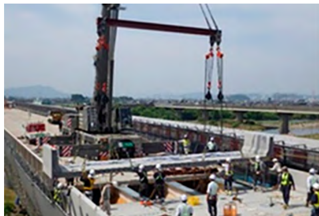
Expressway floor slab replacement works
