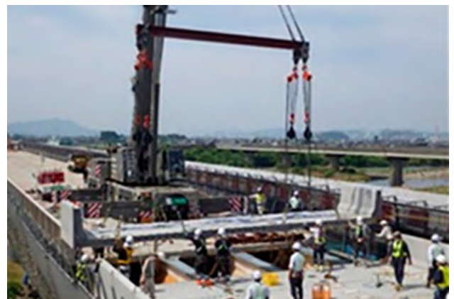
Expressway floor slab replacement works
