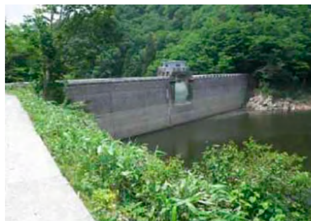
Nakatsu Dam (photo from the official website of Tottori Prefecture)
