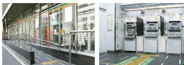
Ramps and handrails as well as Braille walkway blocks have been installed at branch entrances and exits as well as ATMs.
