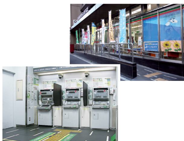
Ramps and handrails as well as Braille walkway blocks have been installed at branch entrances and exits as well as ATMs.
